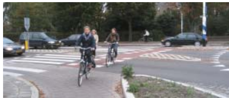
Cyclists and pedestrians at roundabouts in Holland have right-of-way on dedicated paths on the outer edge
